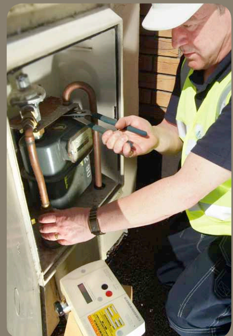
Smart Meter being installed
