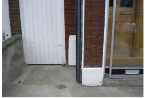
Gas Networks Ireland reinstatement.
