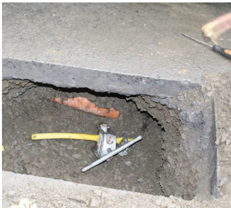
During: Concrete driveway open cut.
