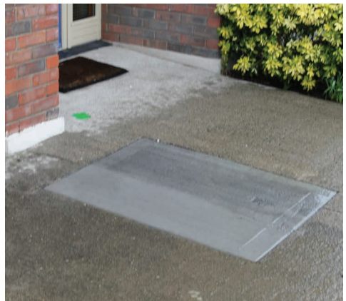
After: Permanent reinstatement – concrete.
