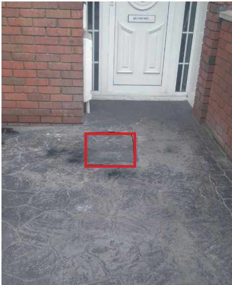
Temporary reinstatement on printed concrete.
