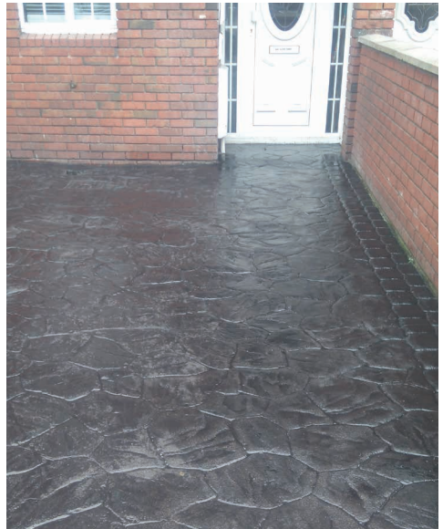
Permanent reinstatement on printed concrete.
